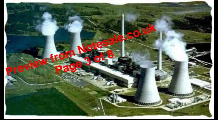
Fission reaction of uranium in nuclear power plants into a very high degree of energy to provide the heating of water vapor. Nuclear power plants convert the energy released from the nucleus of an atom via <u>nuclear fission</u> that takes place in a <u>nuclear reactor</u>. The heat is from the reactor core by a cooling system removes heat and used to generate steam which drives a <u>steam turbine</u> connected to a <u>generator</u> which produces <u>electricity</u>.
